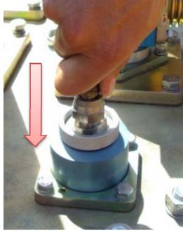
1. Release any pressure remaining in the float assembly by unscrewing the sensor lock ring and depressing into the float body. Any excess pressure will release into the tank ullage space.
