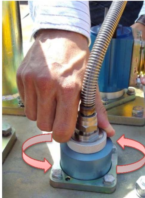
3. Part way through a normal tanker delivery (when tank is above 80% full), depress the test top of the sensor cartridge.
