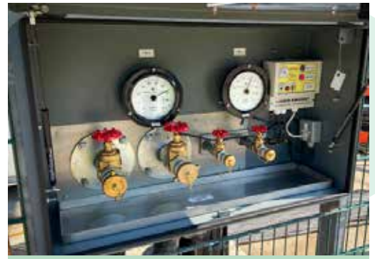
New bulk storage tank filling cabinet with integrated tank gauging & high-level overflow alarm system
