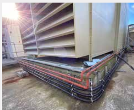
Existing corroding steel pipe with new Doubletrac™ pipework being installed beneath
