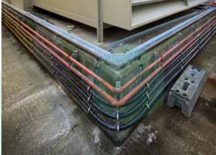
Zero joint pipework runs, fast to install + fire and corrosion resistant. (Note: Original steel pipework is still installed at this point due to the phased installation - you can see the corrosion)
