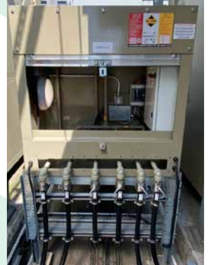
New day tank in-situ with pipework connections finished
