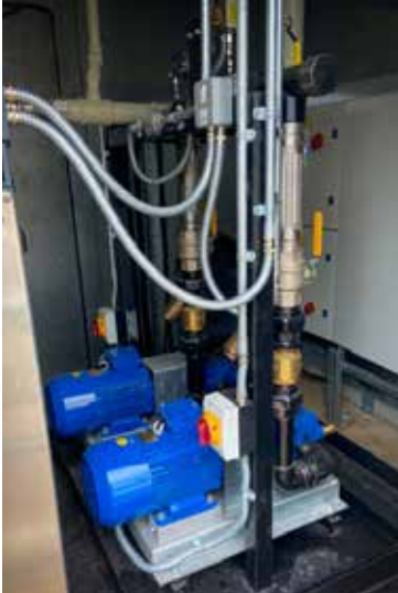
1 of 2 duplex skid mounted pump-sets
