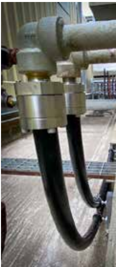
Flexible Doubletrac® pipework system
