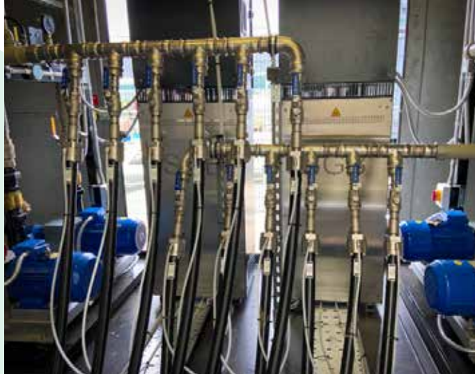
Pump-sets either side of twin day-tank pipework feed manifolds
