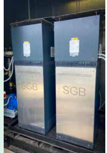
Twin pipework leak detection systems
