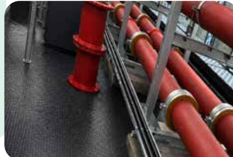
DoubleTrac® pipework secured on cable-tray along the roof-top running towards Generator Day tanks. Zero joint pipework runs, fast install + fire and corrosion resistant.
