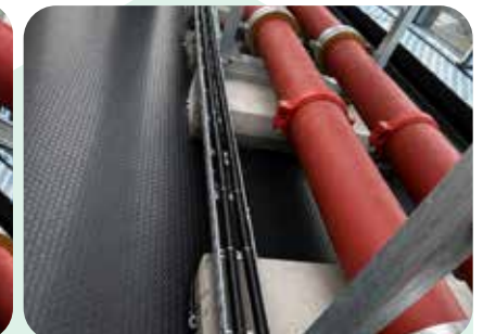
DoubleTrac® pipework secured on cable-tray along the roof-top running towards Generator Day tanks. Zero joint pipework runs, fast install + fire and corrosion resistant.
