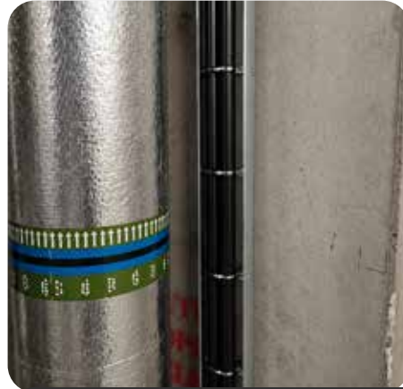
2 X DoubleTrac® pipework runs installed on cable-tray inside internal building service risers. Continuous pipe runs with low 300mm natural bend-radius ensures fast and simple installation when compared to welded steel, with no hot works.
