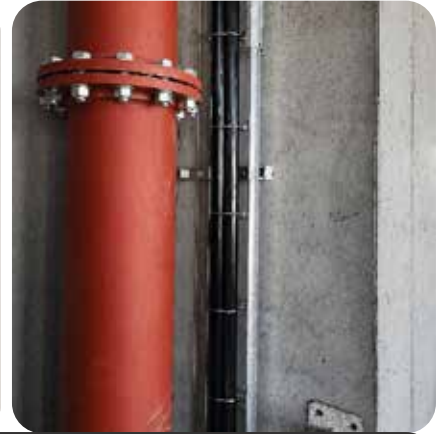
2 X DoubleTrac® pipework runs installed on cable-tray inside internal building service risers. Continuous pipe runs with low 300mm natural bend-radius ensures fast and simple installation when compared to welded steel, with no hot works.
