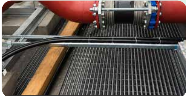
DoubleTrac® pipework exiting service riser onto external roof-top. The natural bend radius of the pipework reduces the need for fittings or joints.
