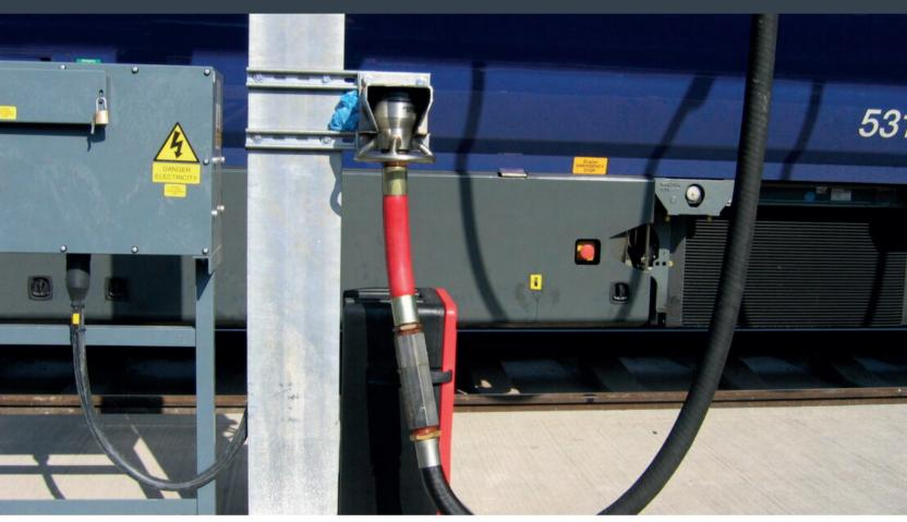
The Rail Flyte Coupling is used for the refuelling of trains in rail service depots. This dry disconnect type coupling has a 1/2" BSP threaded inlet and is designed to fit onto a standard 1-1/2" BSP threaded fuel hose.
