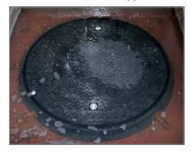
seal. This sealing system has been designed not only to perform from the point of installation but also simple to replace, when required.
